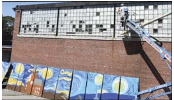
ABOVE: Using a borrowed lift from Wayne Electric and Alarms, Jay Charbonneau of In-House Custom attaches a beam that the panels will be nailed into to cover the broken glass blocks on the south side of the Rogers School in Fairhaven. LEFT: The colorful mural on the addition with the original building towering above. BELOW: Mr. Charbonneau maneuvers the panel into place. Beth David photos.
